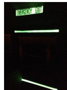
Post-installation: at night – no light
